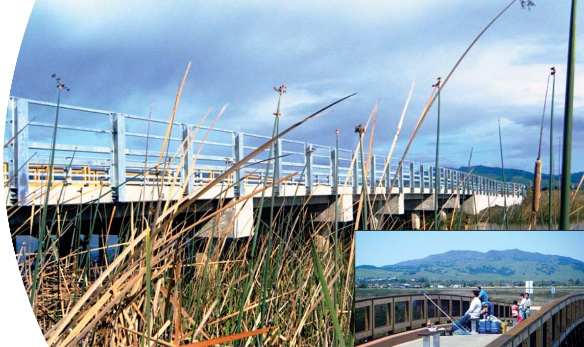
*A new Grizzly Island Road bridge at Hill Slough was built adjacent to the old one-lane timber bridge that was converted to a fishing pier.*
